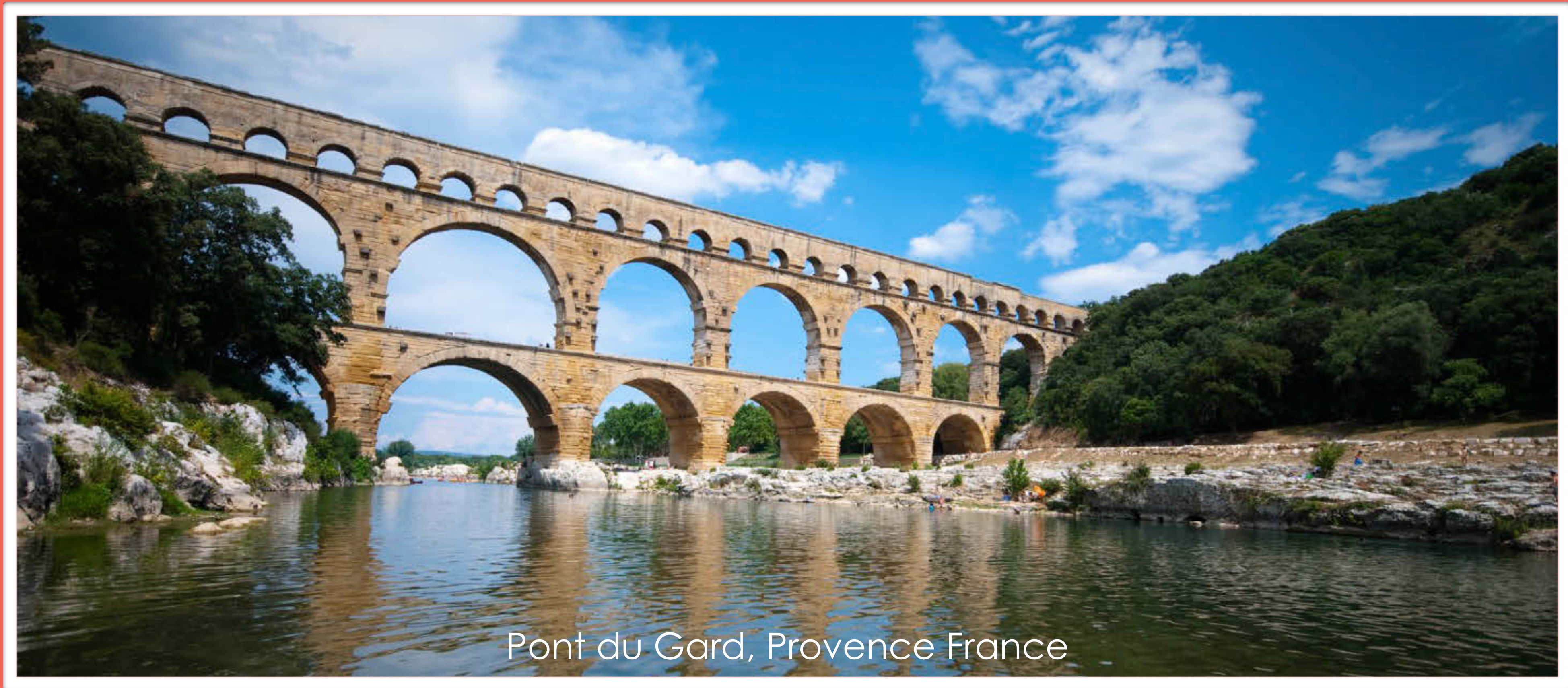
A Roman aqueduct
